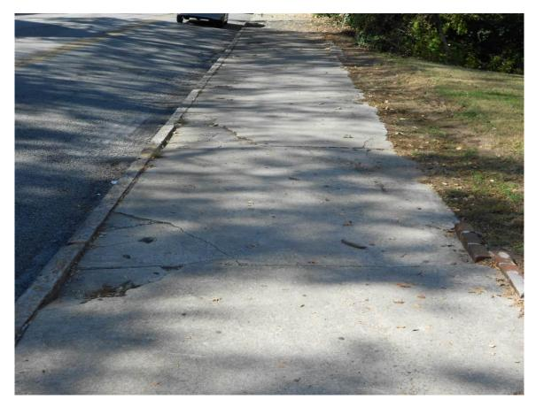
Figure 56. Poor Sidewalk Quality
